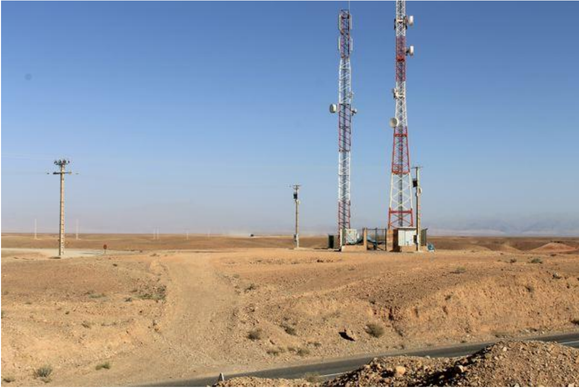
Plate 16-1 Communication towers at the intersection of N10 and the site access road
